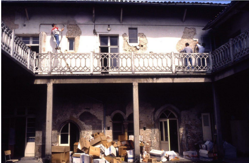
RDC façade EST [avant destruction]
